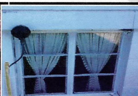
The vent of this regulator is located near a working window. This must be 3ft. away
