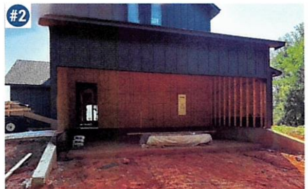
This outdoor unit was placed in a carport with 75 % of the walls closed to vent out
